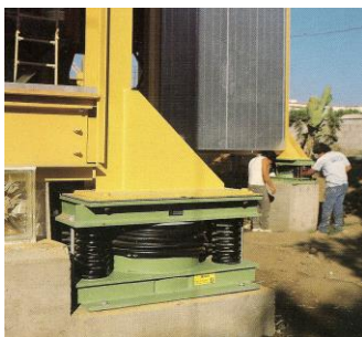
Figure 4. Damper design
