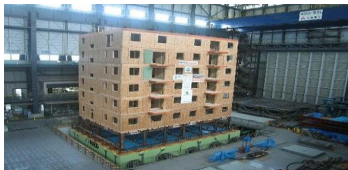
Figure 3. Technology of building construction on a rail platform
