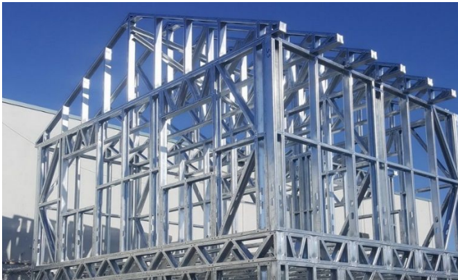
Fig. 1. 3D printing of metal structures company, LifeTec Construction Group
